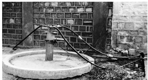
Fig. 3. Hand pump equipped with jet pump in Mandimirja Kha village, Fatehpur Sikri block.
