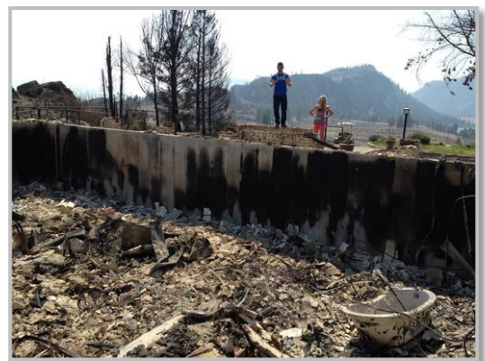
Damage from the 2014 Pateros wildfire.
